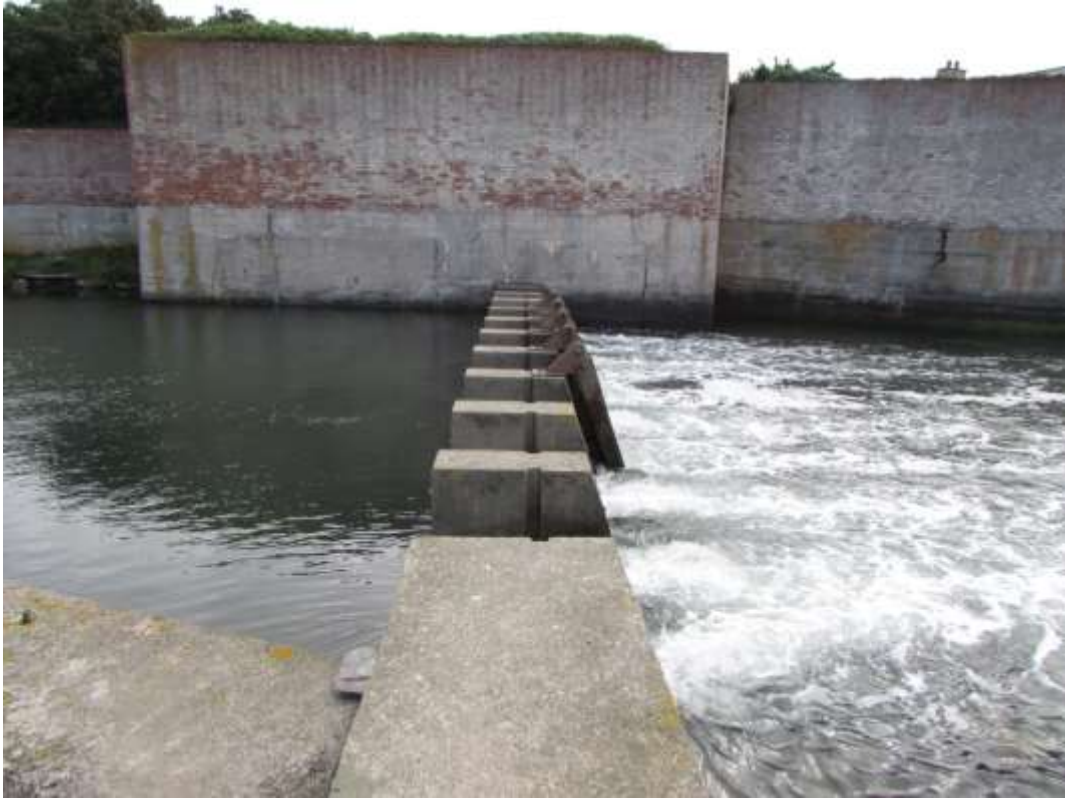
Figure 35. Peak outward flow over the weir, approximately 1 hour after the time of high water, 13.45 on 14 August 2018
