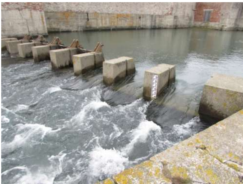
Figure 31. Onward flow across the weir at time of maximum flood tide stage rise, 11.00 on 14 August 2018
