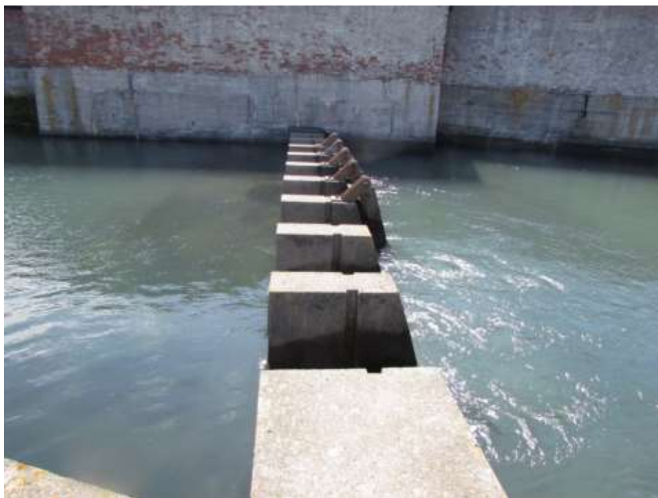
Figure 34. The beginning of outward flow over the weir, just after the tide started to ebb, 13.00 on 14 August 2018
